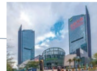
Shenzhen FA Center MITSUBISHI ELECTRIC AUTOMATION (CHINA) LTD.
