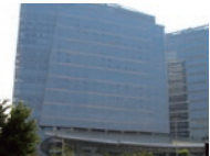
Guangzhou FA Center MITSUBISHI ELECTRIC AUTOMATION (CHINA)LTD.
