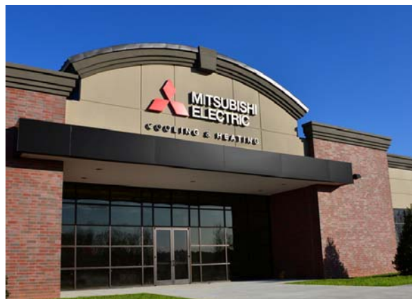
New Cooling & Heating Division HQ of Mitsubishi Electric US, Inc.
