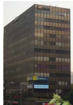
New Indonesia FA Center at PT. Mitsubishi Electric Indonesia.
