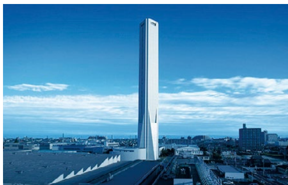
SOLAÉ elevator testing tower
