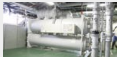
Centrifugal Refrigerating Machines Centrifugal refrigerating machines were updated for air-conditioned, cold water manufacturing to cut power consumption by 9%.
