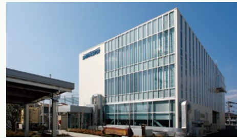
Shirasagi Denki Kogyo Co., Ltd. head office building
