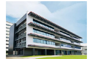
ZEB testing facility "SUSTIE"
