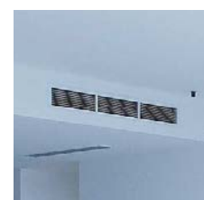
The living room vent of an indoor unit for a condominium
