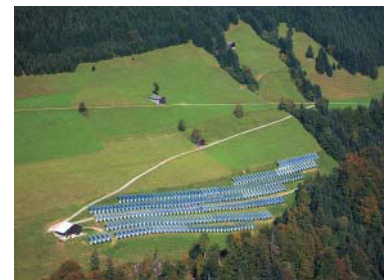
Fig. 4 Installation sample of small-scale power generation
