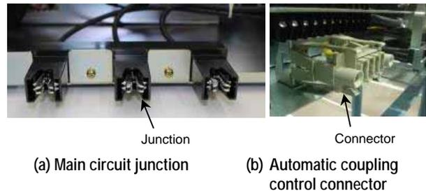
**Fig. 3 Main circuit junction and automatic coupling control connector**
