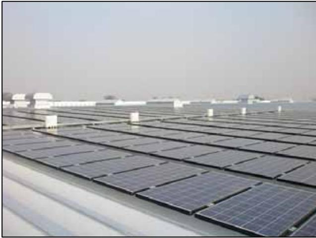
Fig. 1) 51 kW PV system on the warehouse roof (above)
