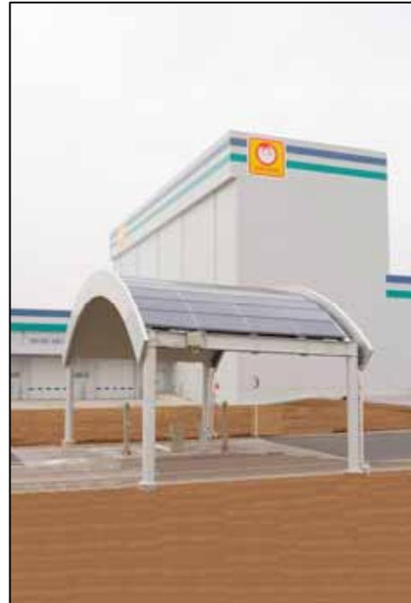
Fig. 2) 11 kW PV system on the main gate arch (right)
