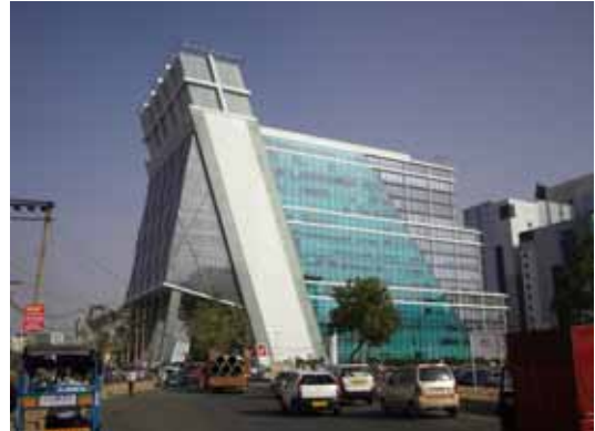
Office building that houses Mitsubishi Electric India Gurgaon Head Office
