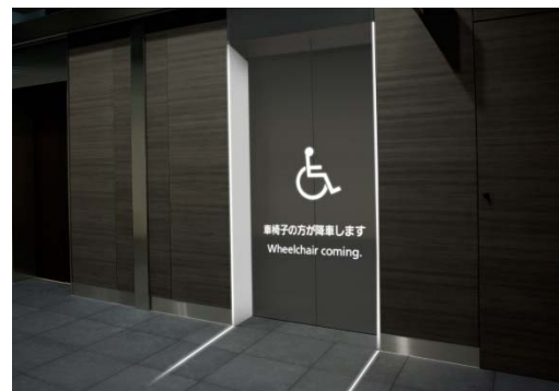
Guidance projected on elevator door
