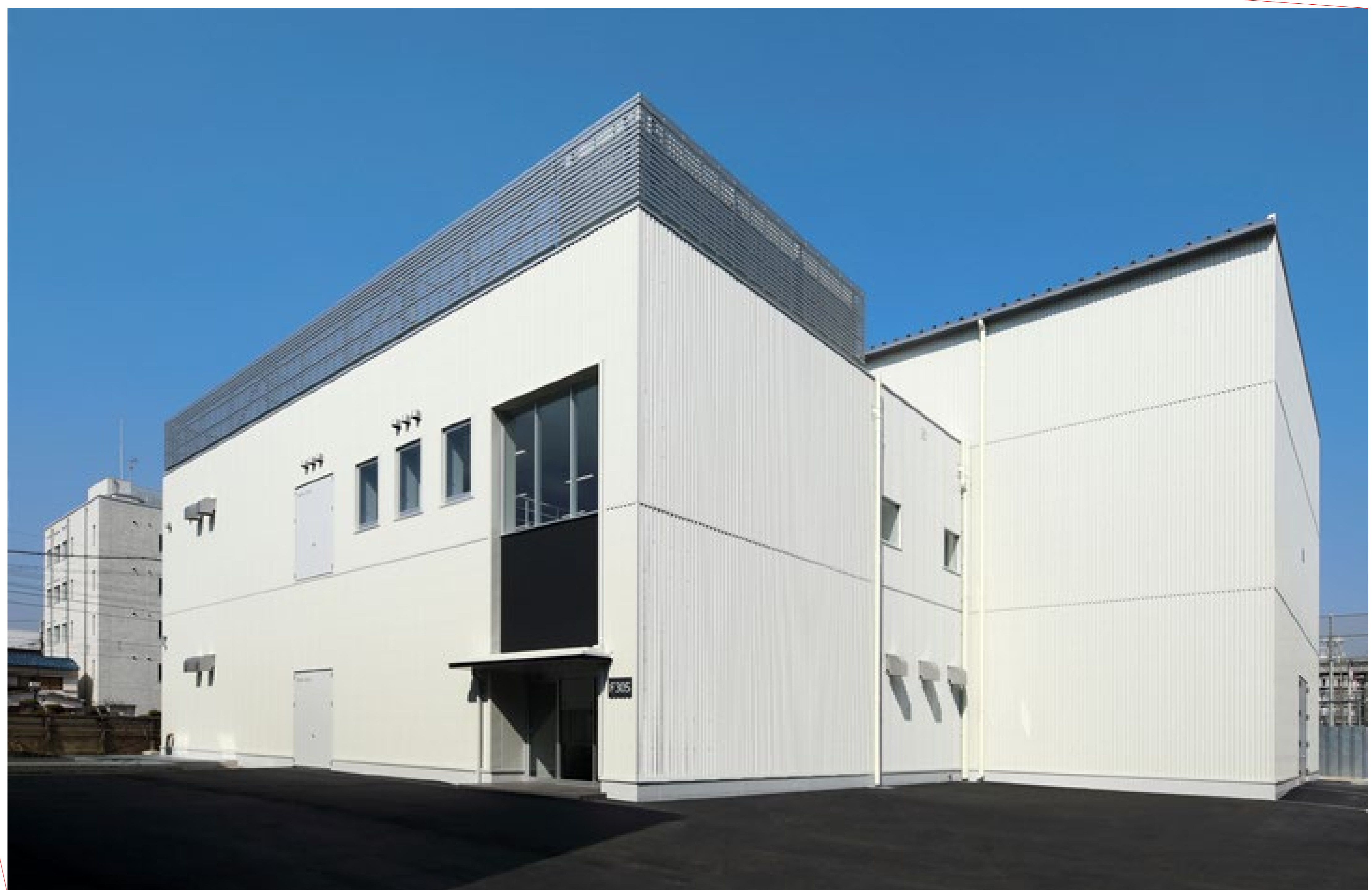
HVDC-Diamond® Verification Facility
