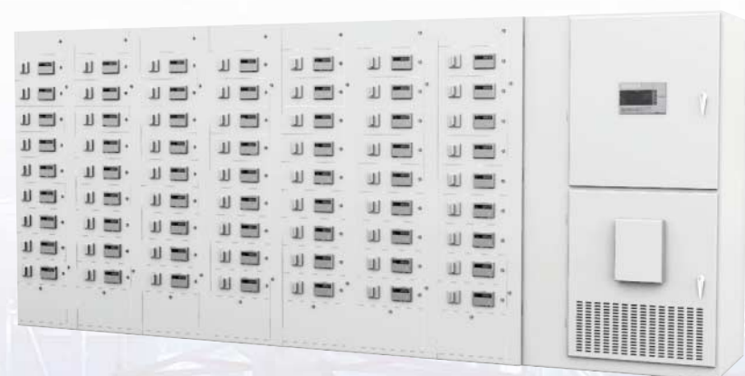
Figure 1-1 AL-P and Motor control center
