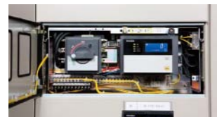
Unit front view
