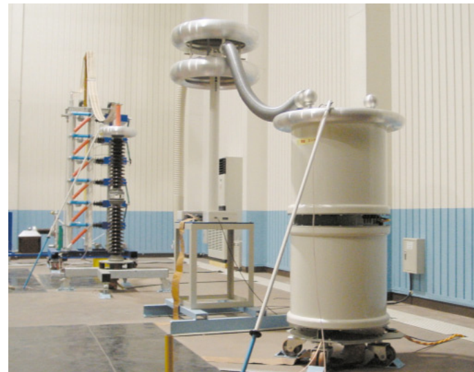
Dielectric test cell
