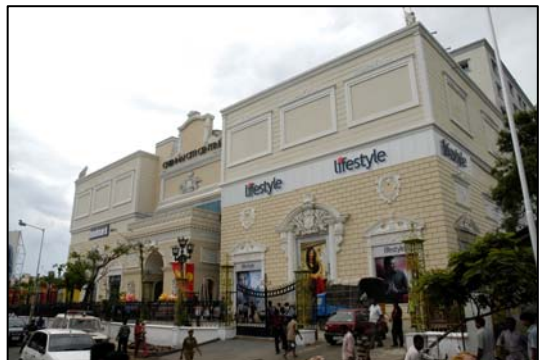
Chennai Citi Centre, location of Mitsubishi Elevator ETA India Private Limited
