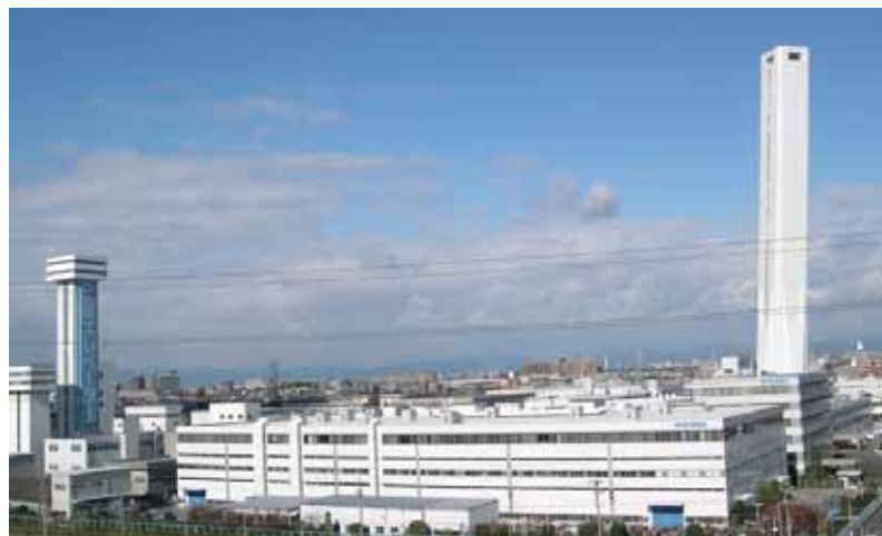
Mitsubishi Electric's Inazawa Works
