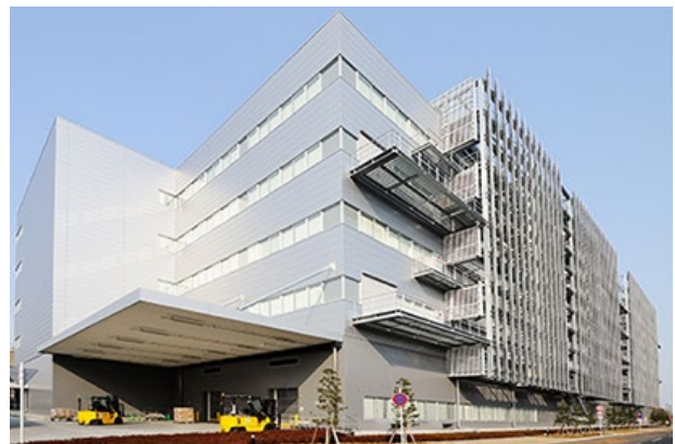
The latest E4 production site harnessing e-F@ctory technologies
