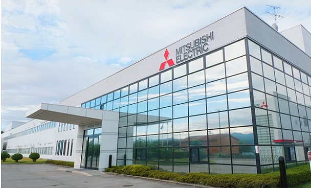
The Iida Factory is a production base for domestic ventilation fans, a core product of Nakatsugawa Works
