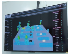
The system visualizes the temperature and humidity inside the clean room. Information from sensors is stored in a database via the MES interface unit. This can be implemented by parameter setting only, making it very easy to use.
