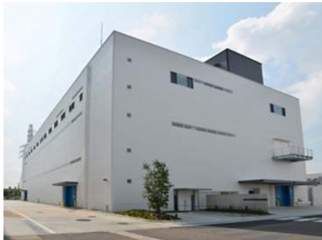
Elevators and Escalators QM center
