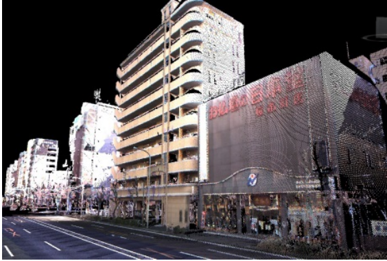
Example 4: Detailed measurement of the building appearance with optional long range or high density laser scanner
