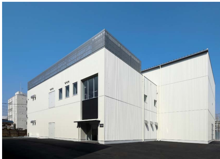
Mitsubishi Electric's new HVDC verification facility
