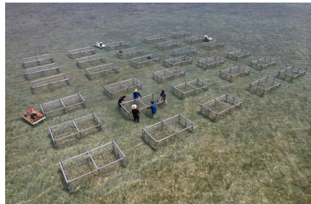
Fences being installed off Takana Beach, Iriomote Island
